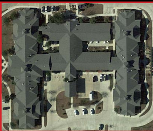
500 East Lake Drive - Taylor - TX
