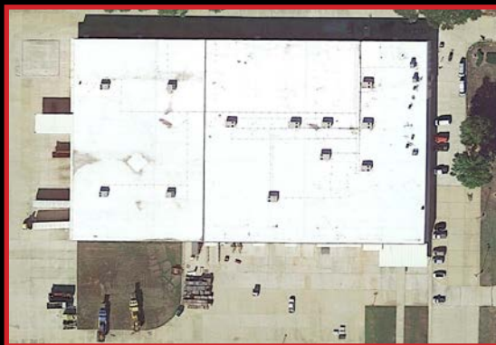
7144 West Park Road - Shreveport - LA
