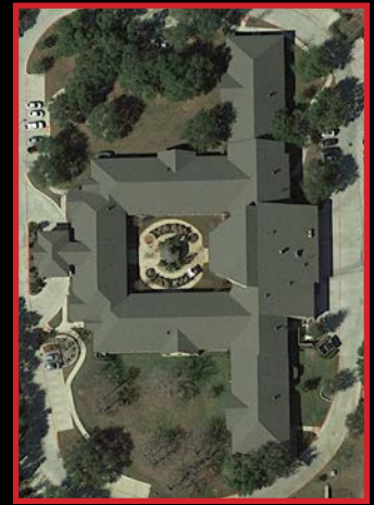
4011 Williams Drive - Georgetown - TX
