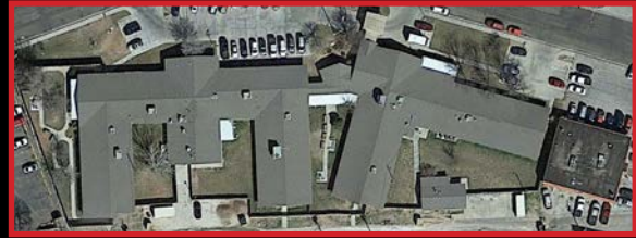
4033 Southwest 51st Avenue - Amarillo - TX
