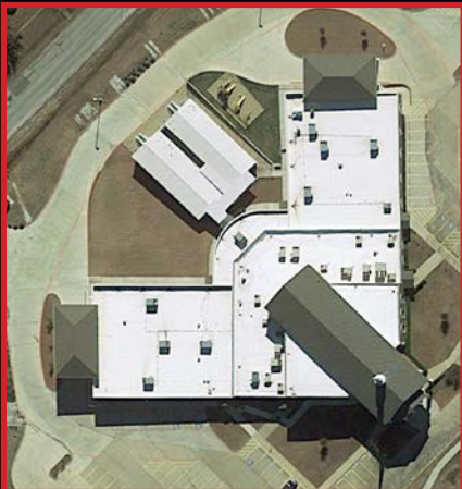
3231 Southwest Wilshire Boulevard - Joshua - TX
