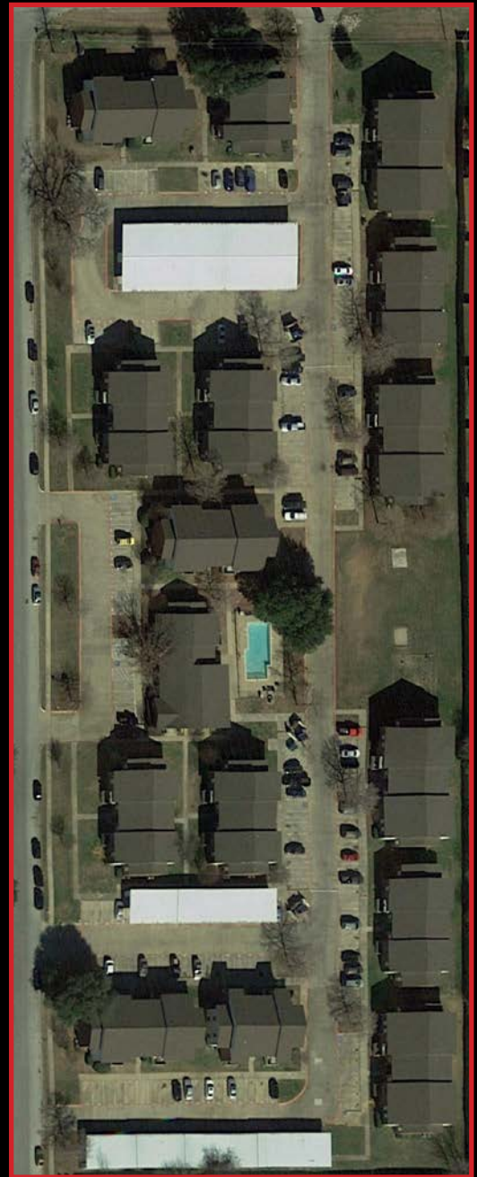
2333 Escalante Avenue - Fort Worth - TX
