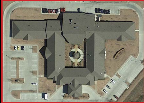
300 Crown Point Blvd - Willow Park - TX
