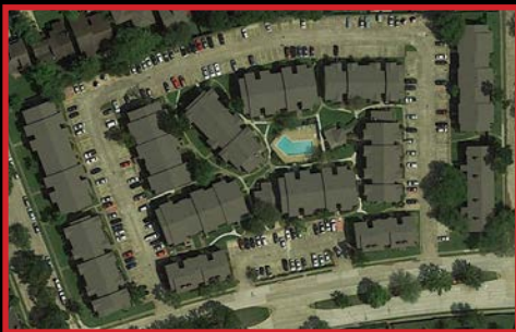
7700 West Airport Blvd - Houston - TX
